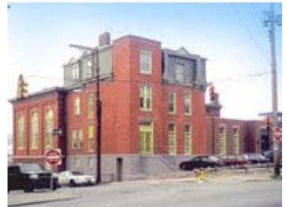
Soho Invention, Inc. before and after renovation
