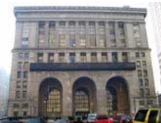
Pittsburgh's City-County Bldg
