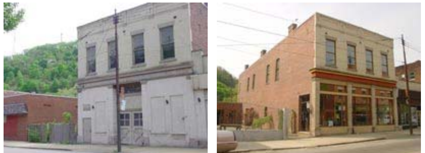
Exterior of James Gallery at 413 S. Main St. - Before and After Renovations
