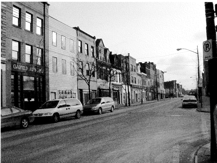
Garfield Street. Clients want to be in a great building in a great neighborhood.
